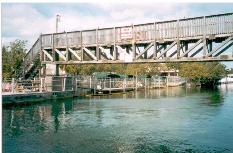
Figure 6.3 View of Study Area from Canal
