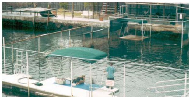
Figure 6.13 Chain Link Fenced Enclosures
