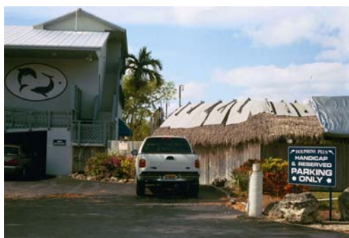
Figure 6.9 Front of Study Site Property
